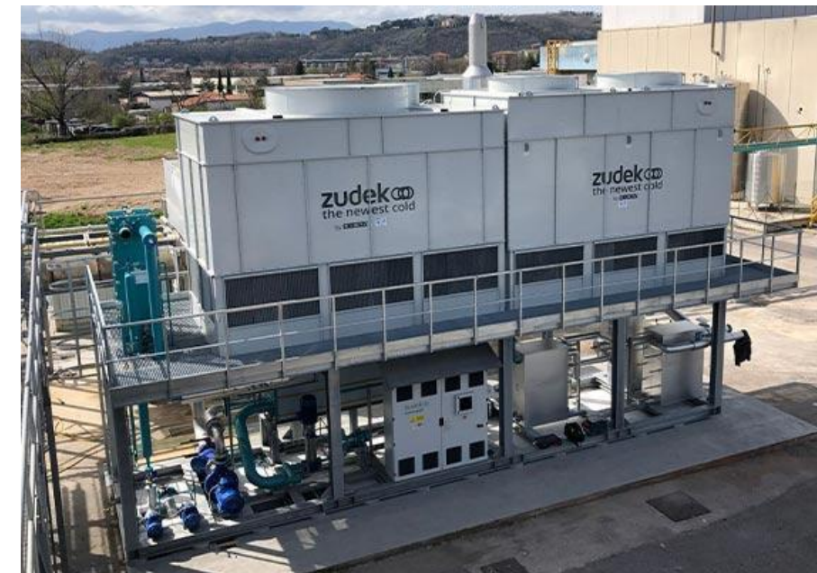
Zudek Srl, Enermatik ammonia-water absorption chiller
