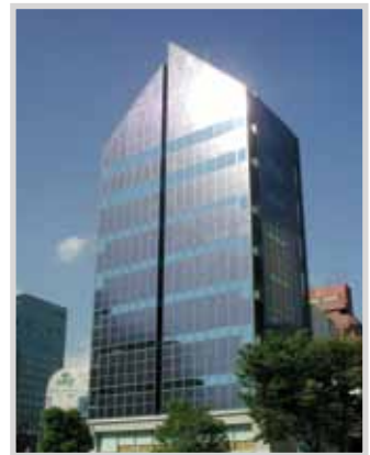
PV system integrated in a facade
