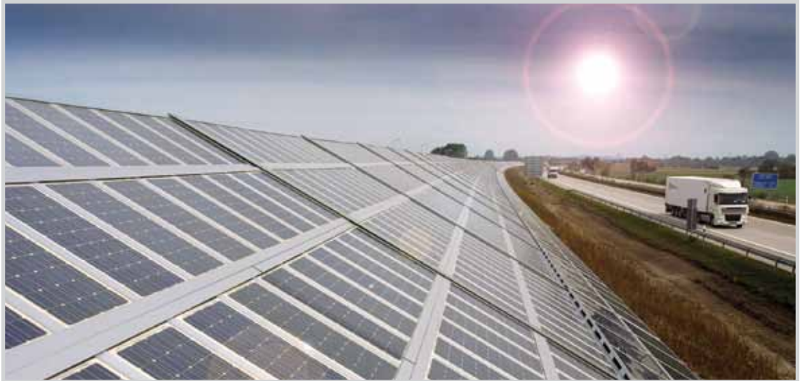
Photovoltaic sound barrier along a motorway
