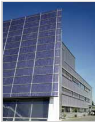
PV system integrated in a facade
