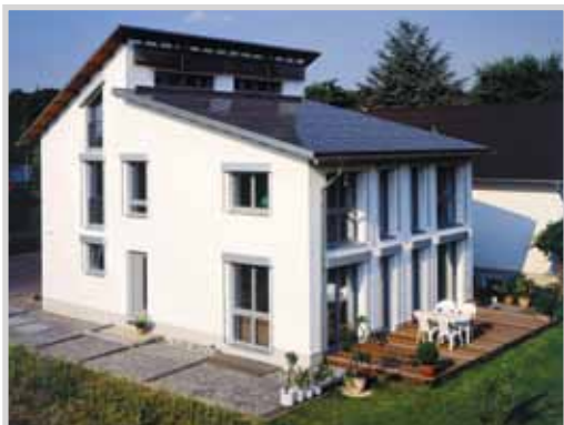
Photovoltaic system integrated on the roof of a house, Germany
