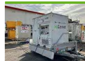
Off-grid construction site
